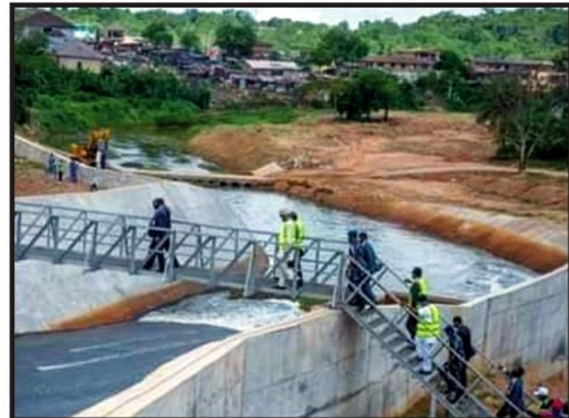
Improved Eleyele Water Dam
