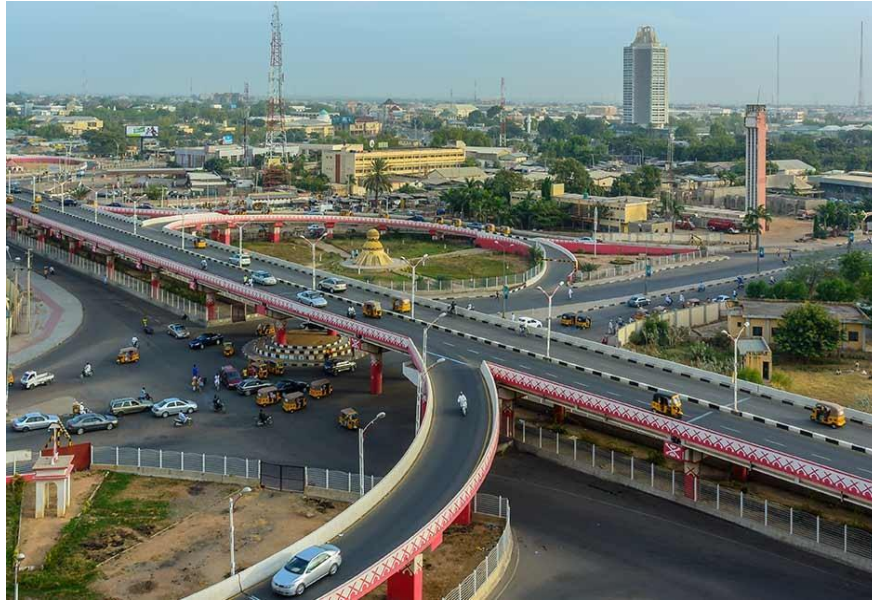
Murtala Mohammed Flyover Kano
