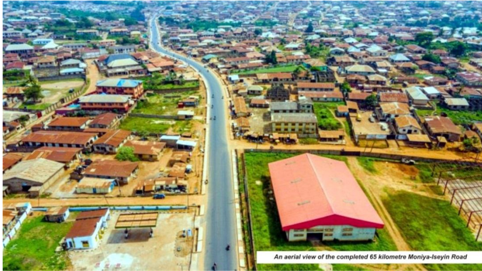
An Aerial View of the completed 65 kilometres Moniya-Iseyin Road
