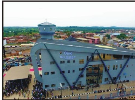
Bus Terminal at Ojoo
